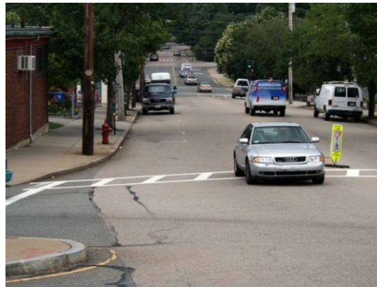
Lexington Street: Potential location for curb extensions
