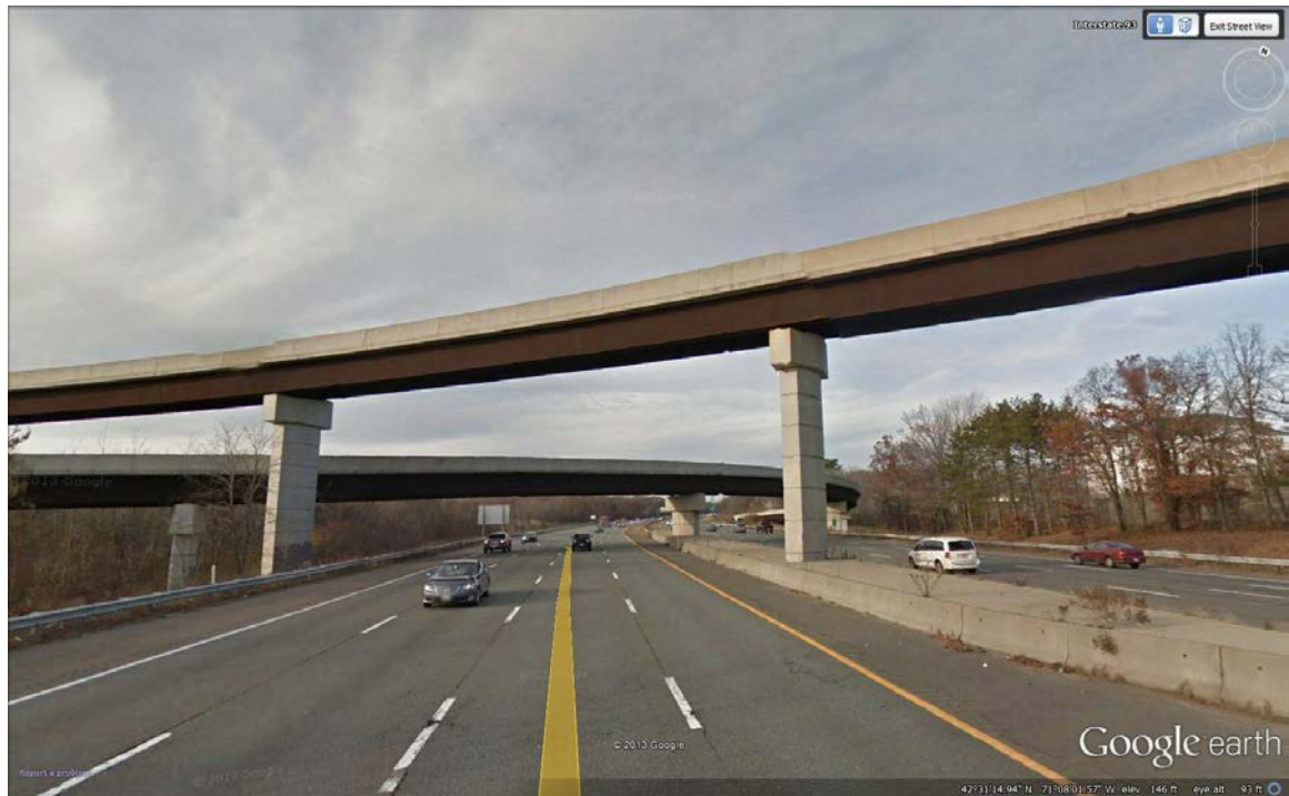
FIGURE 14 Interchange 37C View Looking North in the Southbound Lanes
