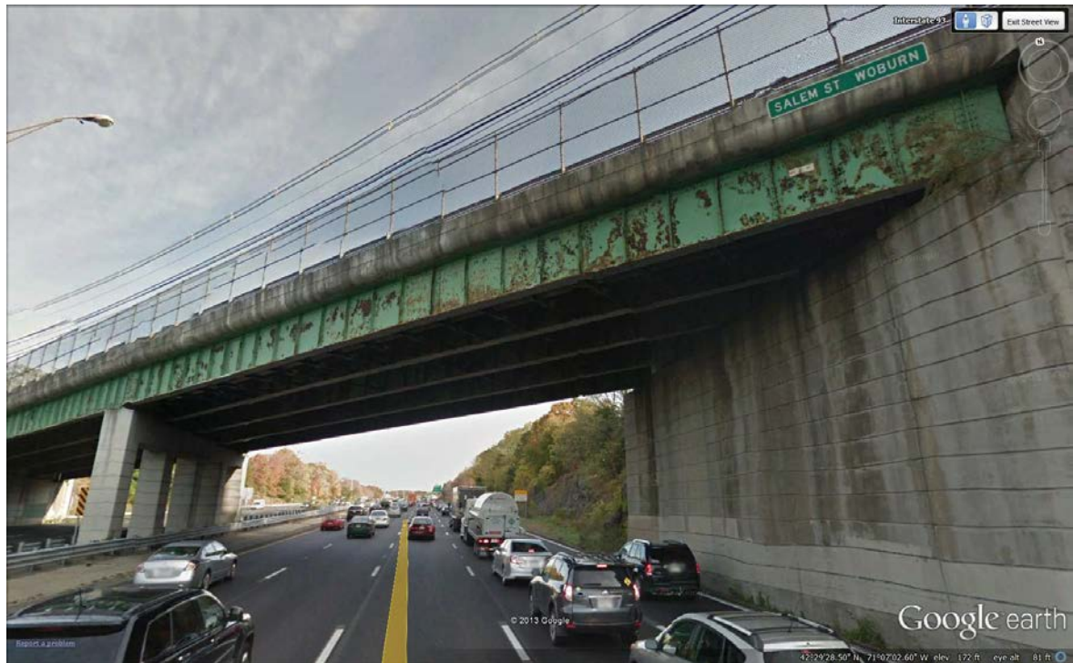
FIGURE 13 Salem Street Bridge View Looking North in the Northbound Lanes
