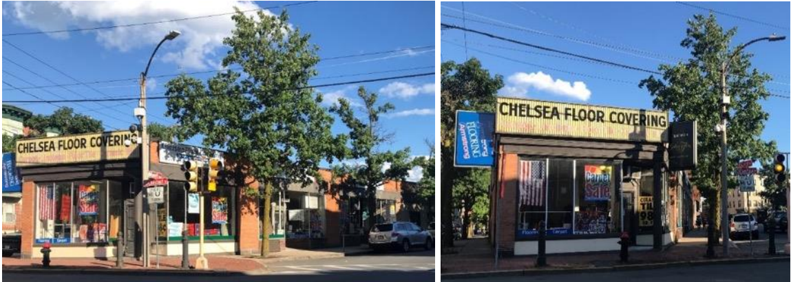
Figure 5 Southeast Corner of Intersection: Chelsea Floor Covering Company
