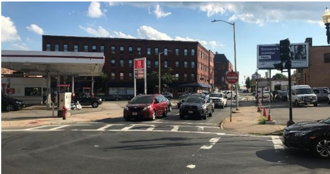
Figure 5 Wide Curb Cuts on Liberty Street Intersection Approach
