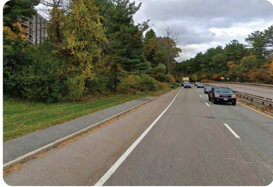
Gap in sidewalk network near Water View Terrace at Framingham Apartments
