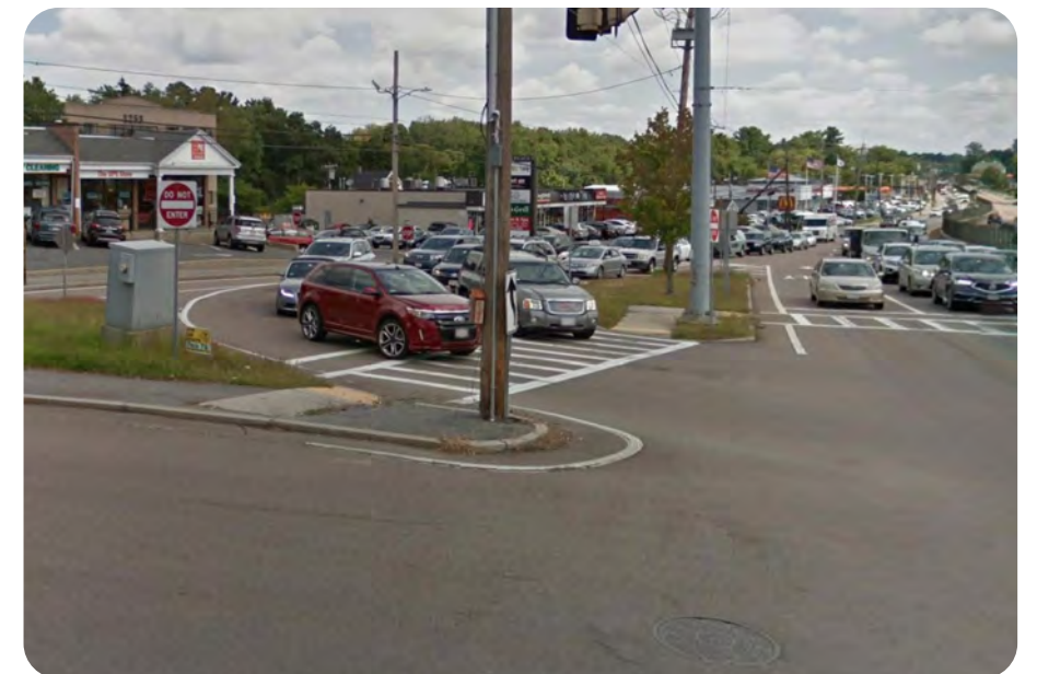
Lack of pedestrian signals and pushbuttons on Temple Street
