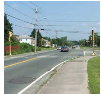
The pedestrian signal phase is too short for the long crosswalks at this intersection.
