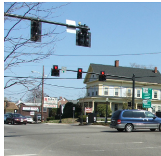
This intersection was reconstructed in 2002.
