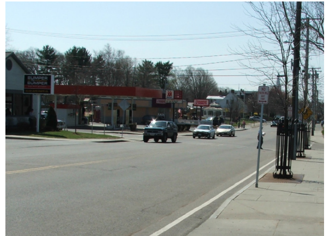
South Franklin Street, looking south
