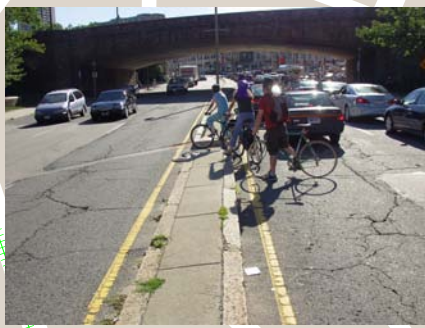
Lack of safe crossing
