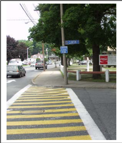
Ladder Style with Parallel Bars Concord and Clinton Streets, Framingham
