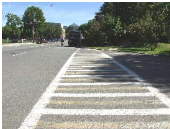
Long crosswalk on River Road at Brookline Avenue.
