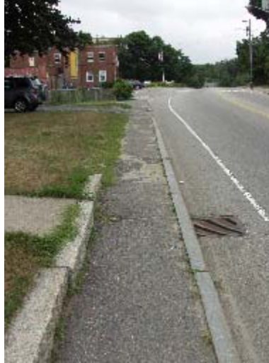
A narrow sidewalk leading to the Teen Center
