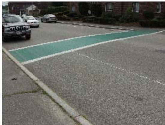
Curb ramp and extension are needed on Broad Street
