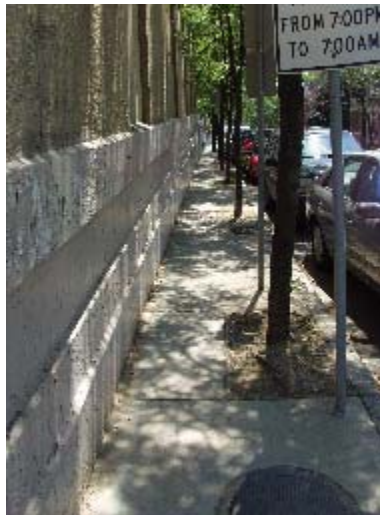
Very narrow sidewalk along Beacon Street (but keep the trees!).
