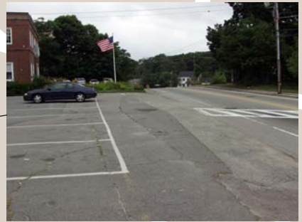
No separation between the street, sidewalk, and parking lot
