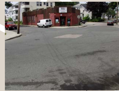
Lack of crosswalks
