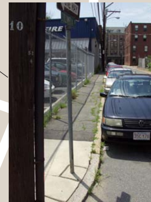
Narrow, obstructed sidewalk
