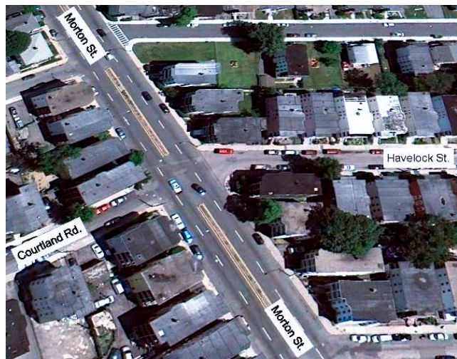
Morton Street at Courtland Road and Havelock Street
