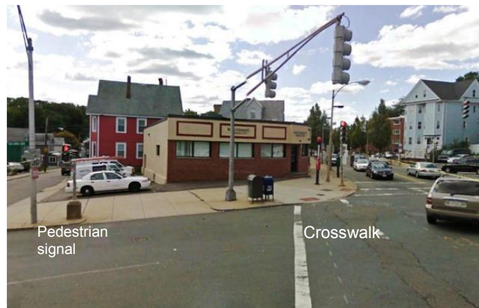
Pedestrian signal not aligned with crosswalk
