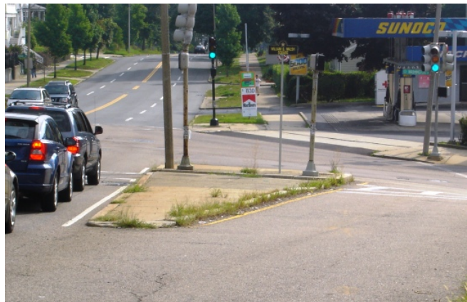
No object marker (OM1-2) installed at the approach of the triangular island
