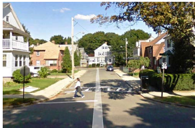
Gallivan Boulevard at Huron Circle: Curb ramps and crosswalk are not aligned to allow pedestrians to stay within the bounds of the sidewalk and the pedestrian desire line.
