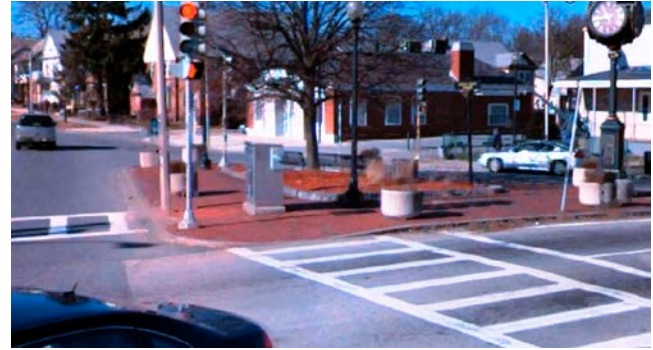
Gallivan Boulevard and Granite Street/Adams Street: Choke points that narrow the effective sidewalk width, such as mailboxes, utility poles and equipment, and landscaping.
