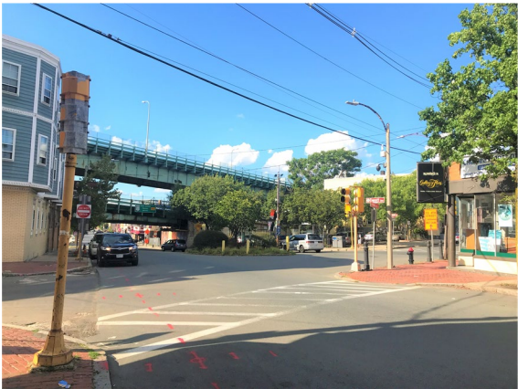
Figure 6 Marked crosswalk on Everett Avenue across southern leg of the intersection.
