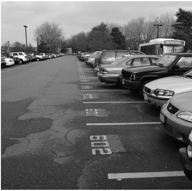
MBTA PARK-AND-RIDE LOT AT OAK GROVE STATION
