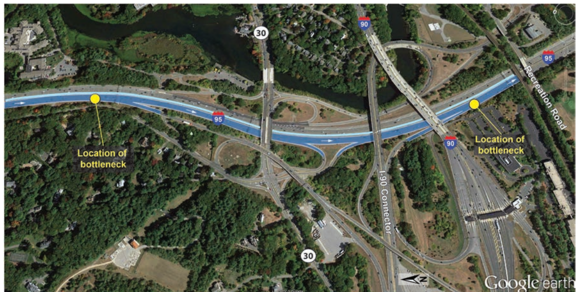
MassDOT is implementing recommendations from an MPO-supported study to address bottlenecks on Interstate 95 southbound between Exit 25 and Recreation Road in Weston. [Photo: Google Earth]
